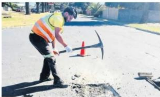
A City worker fixing a pothole.
